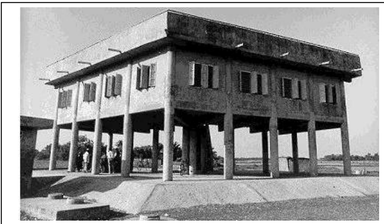
A cyclone shelter in Bangladesh
